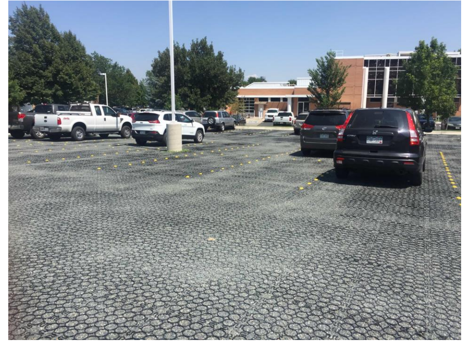
City of Fort Collins, Colorado
