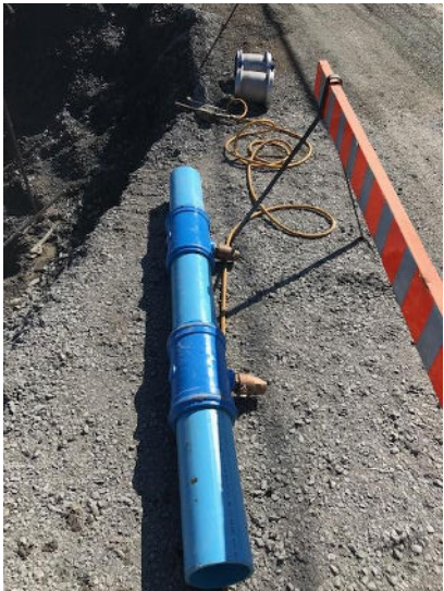
Materials used for the repair
