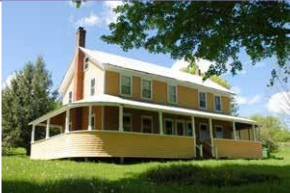
PRENTICE HOUSE: 208 NORTH SUTTON ROAD
